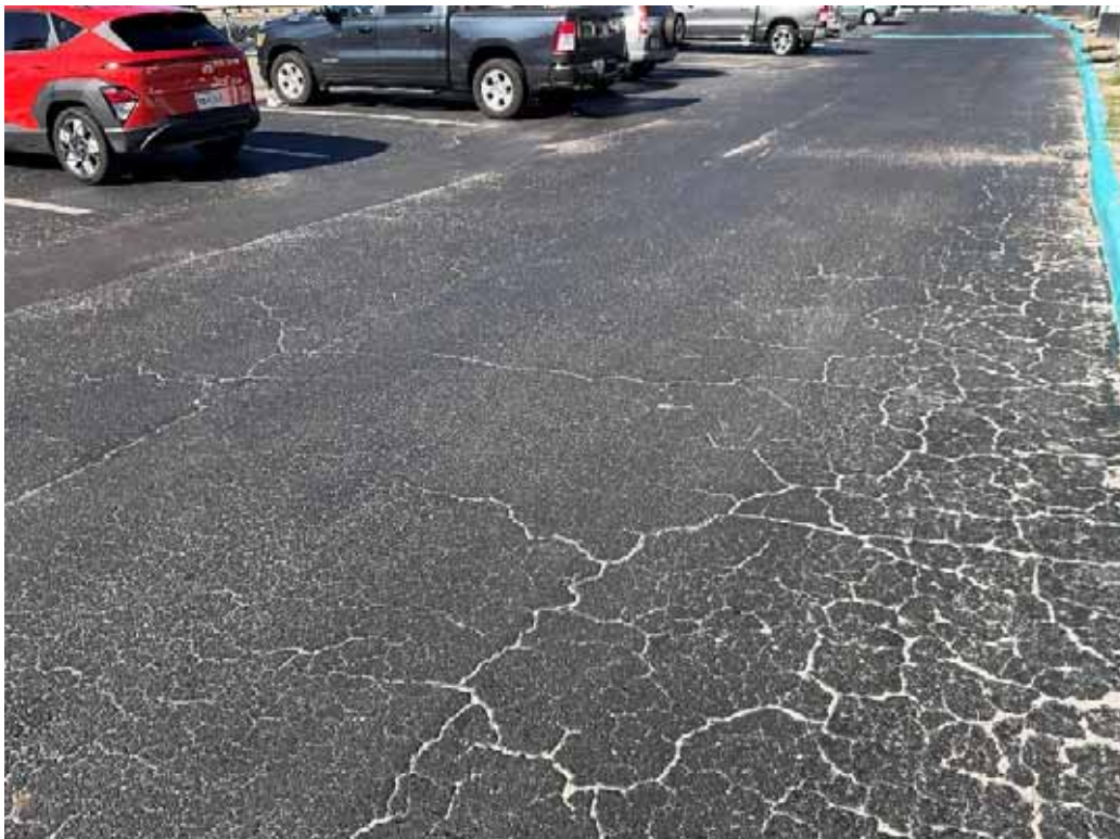
Pavement, Asphalt - Parking Lot
