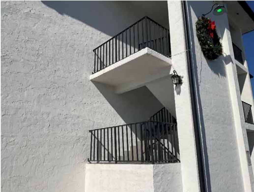
Bldg B Stairway Railing
