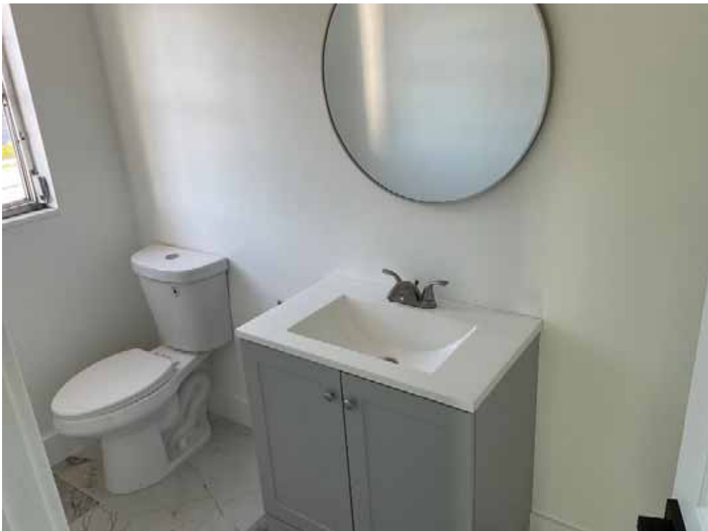
Bldg A Billiards Room Restroom
