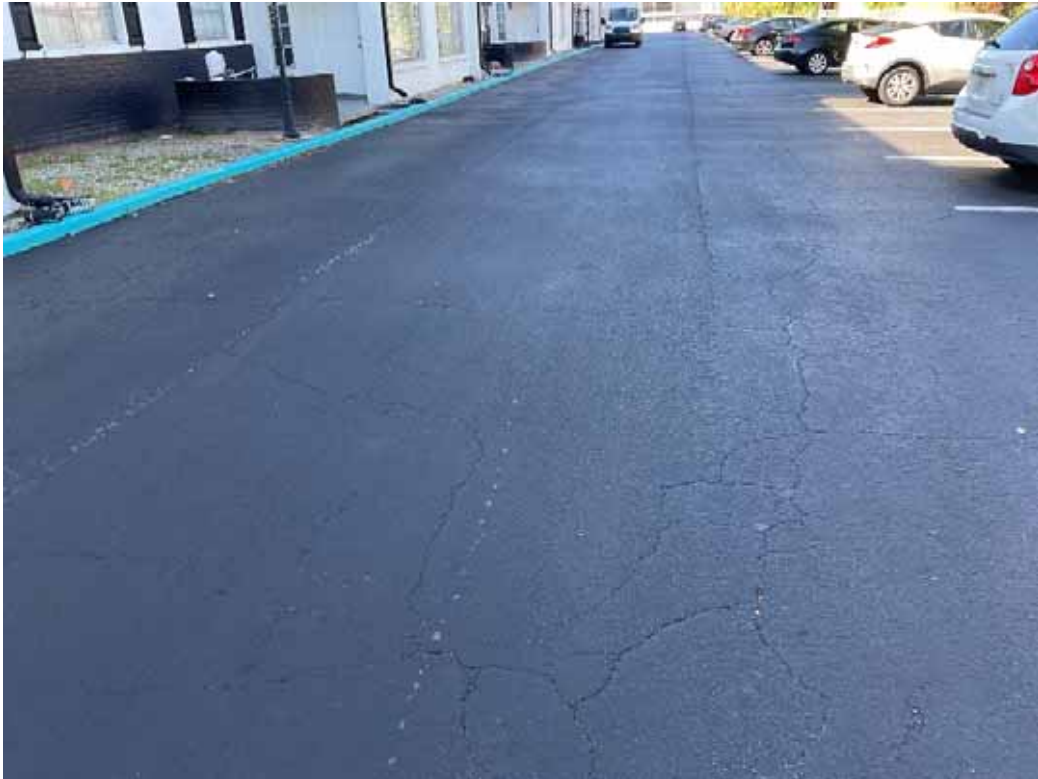
Pavement, Asphalt - Parking Lot
