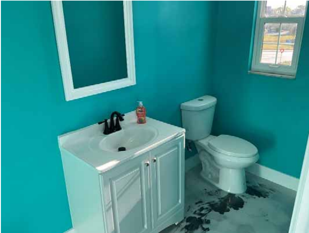
Bldg A Card Room Restroom (1 of 2)
