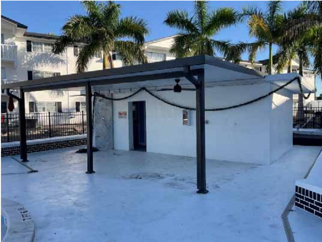
Pool Restroom Bldg
