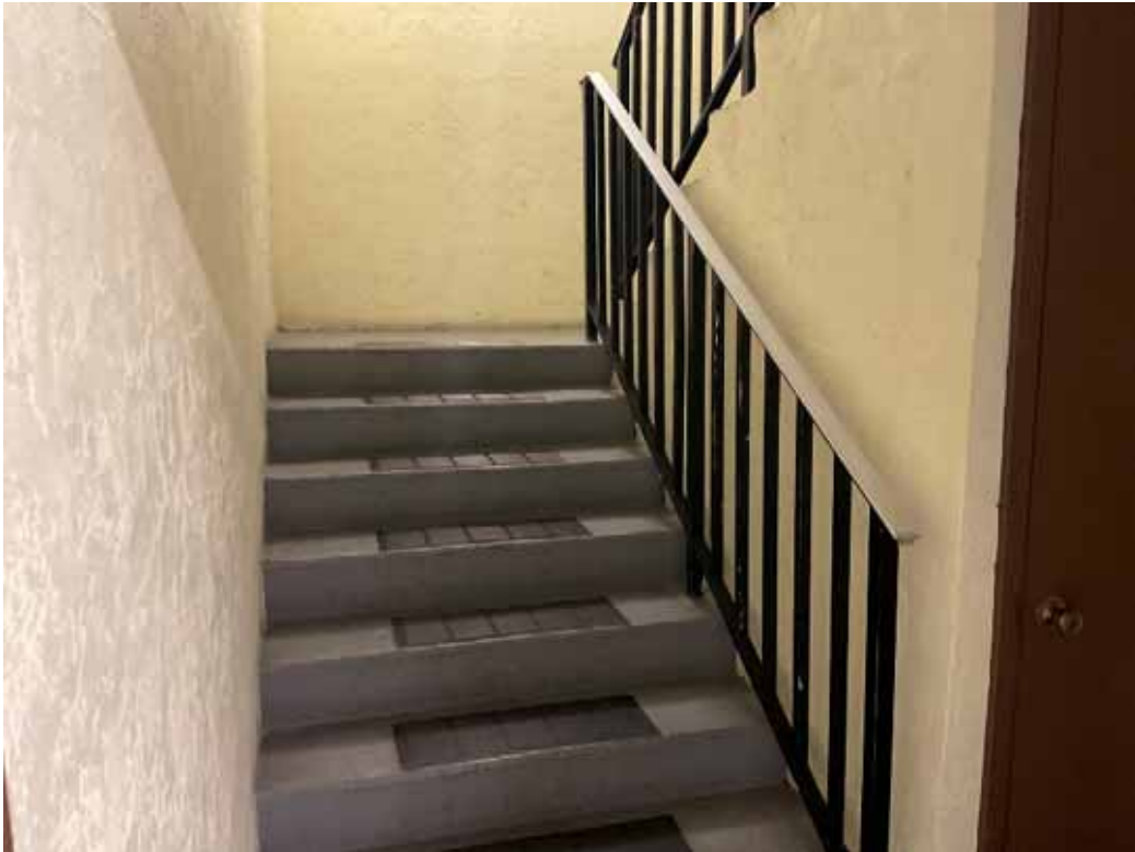
Bldg A Stairwell
