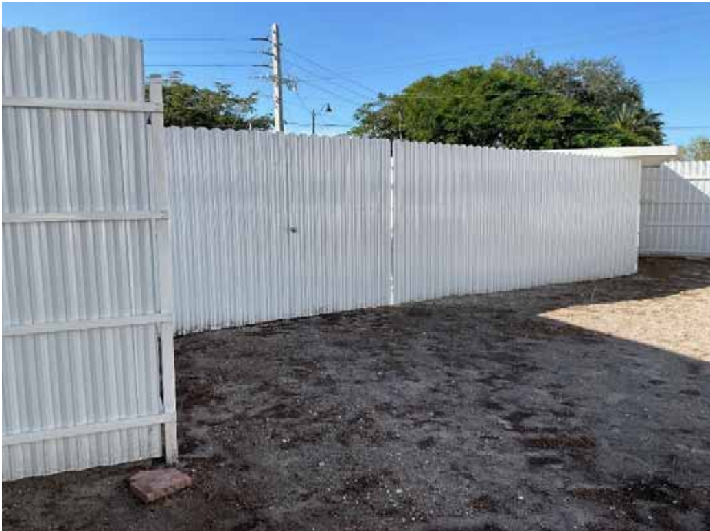
Recreation Area Fence
