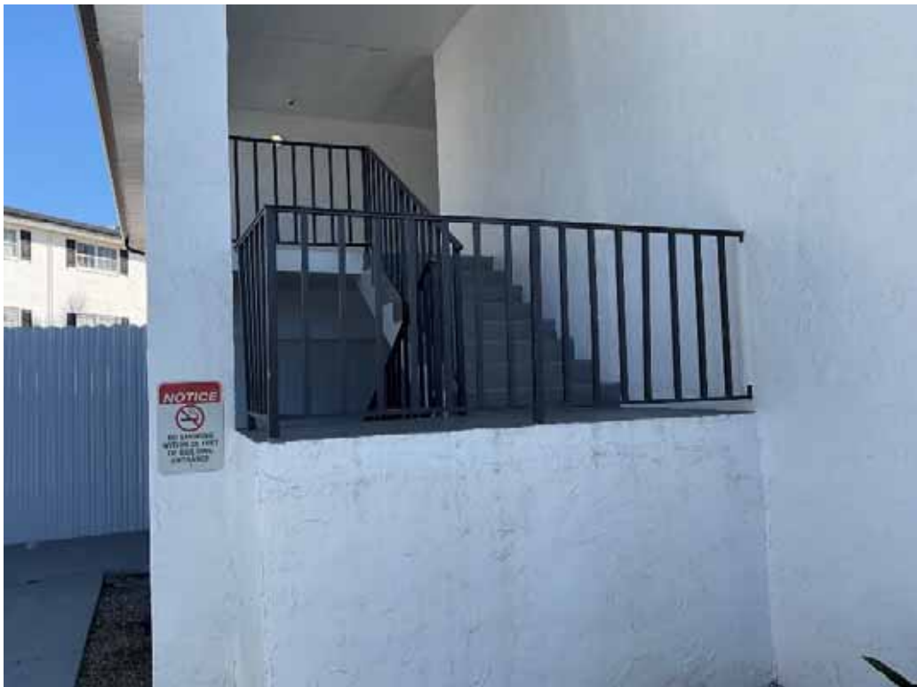
Bldg A Stairway Railing
