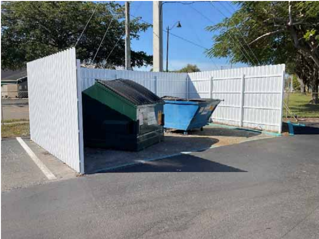
Bldg A Trash Enclosure
