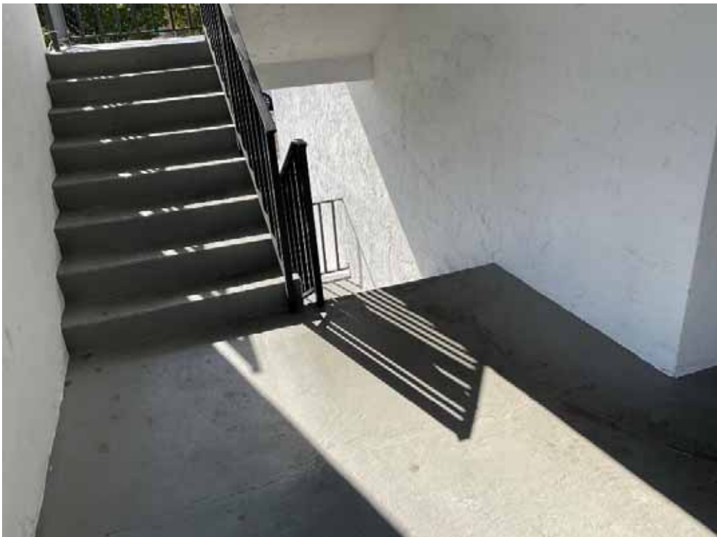
Bldg B Stairway
