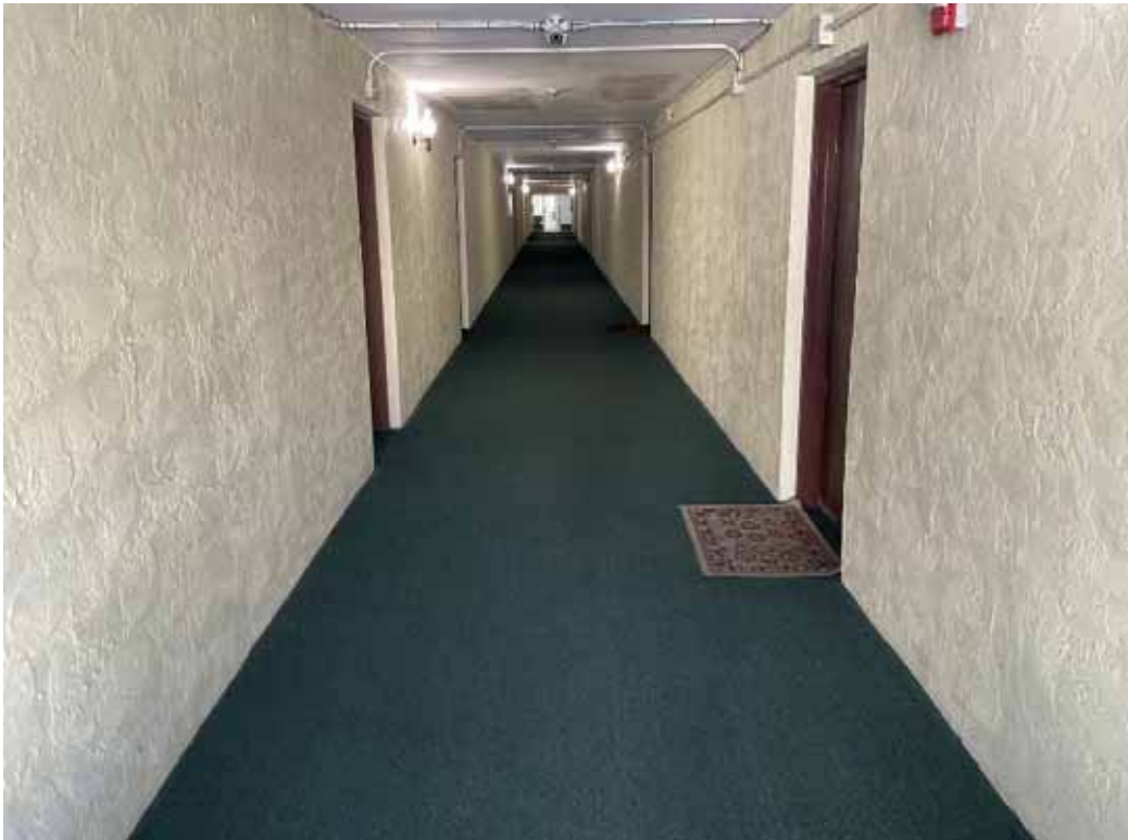
Bldg A Hallway - 2nd Floor
