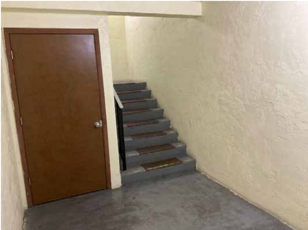
Bldg B Stairwell
