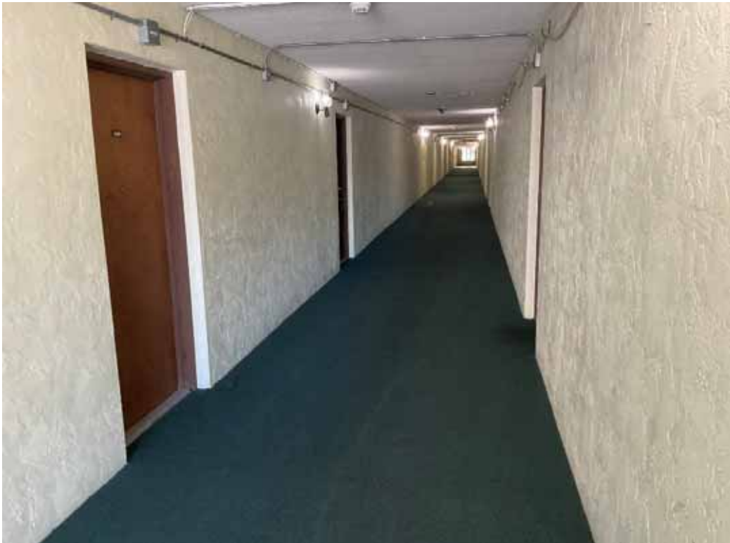
Bldg B Hallway - 1st Floor
