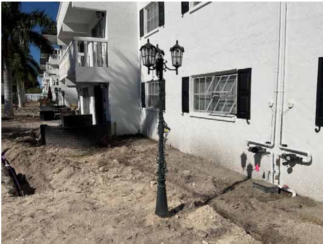
Light Pole & Fixture - Recreation Area
