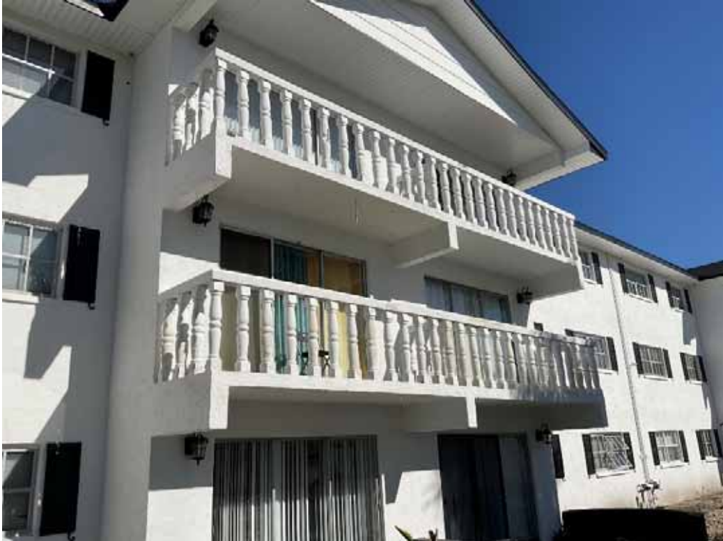
Bldg B Balconies
