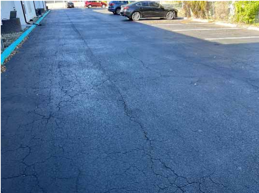
Pavement, Asphalt - Parking Lot
