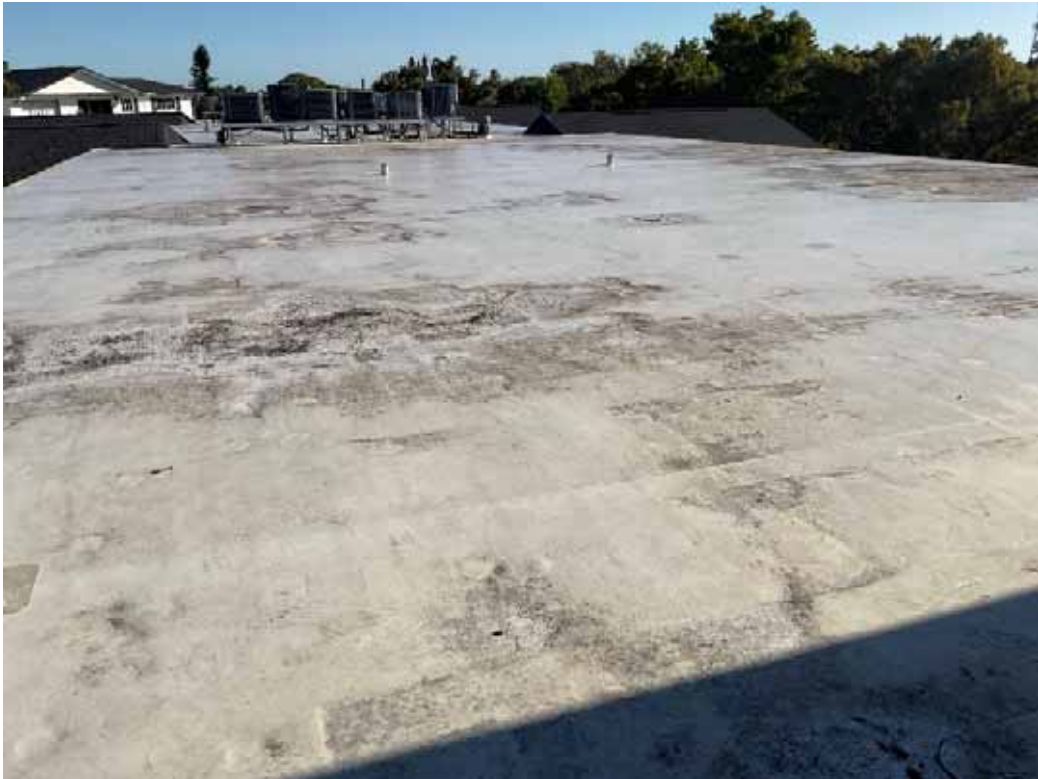
Bldg A Roof
