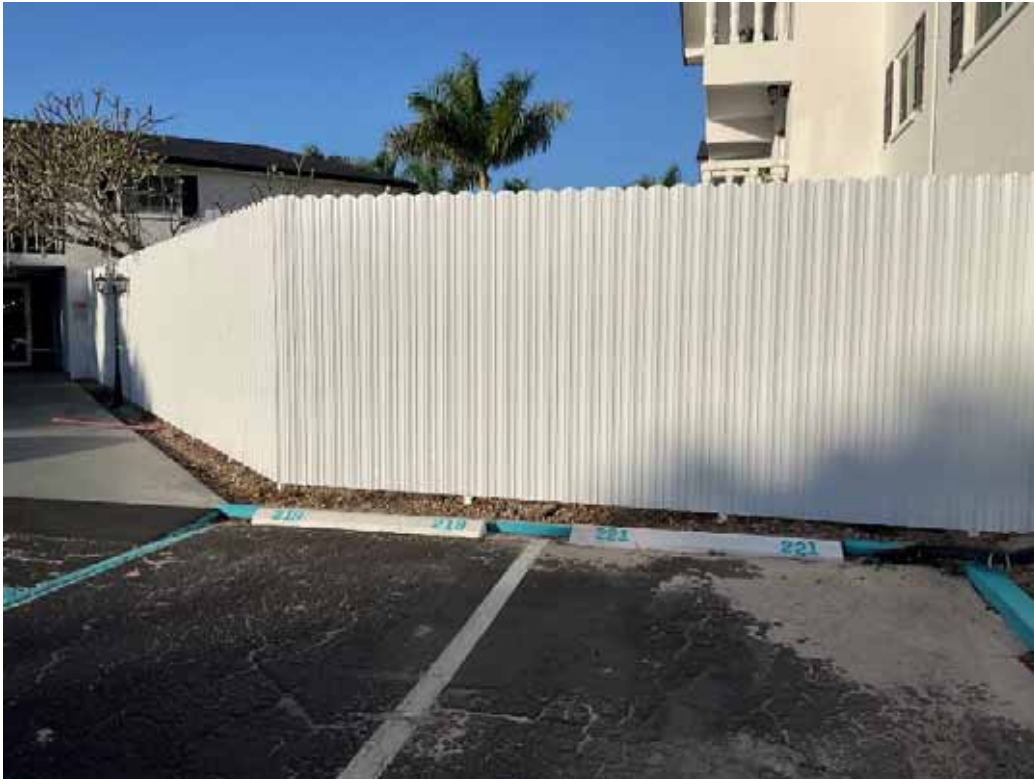
Recreation Area Fence
