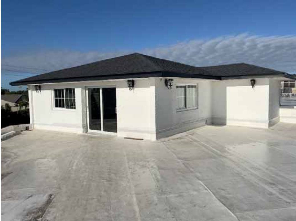
Bldg A Card Room Exterior (1 of 2)
