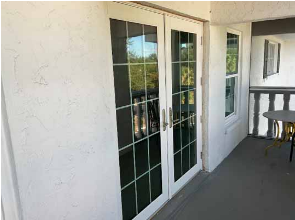
Bldg B Window & Doors - Library
