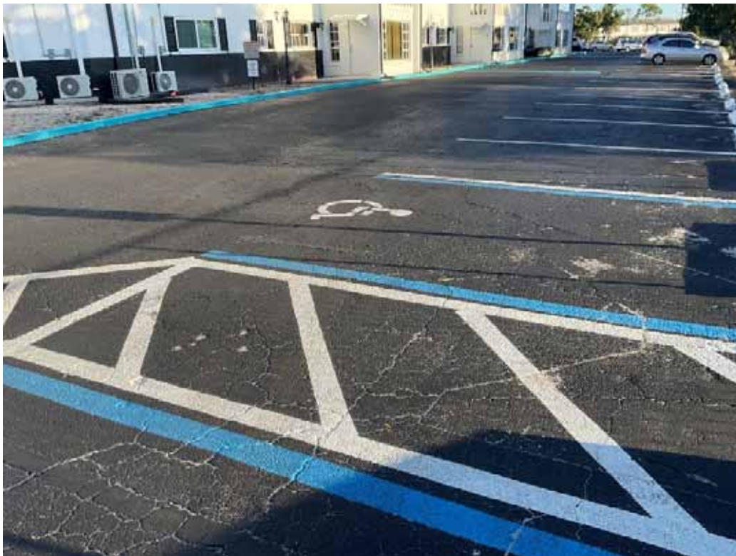
Pavement, Asphalt - Parking Lot
