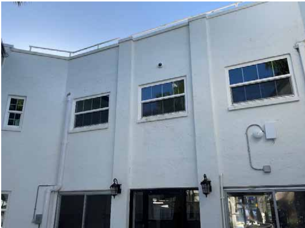
Bldg A Windows - Community Room
