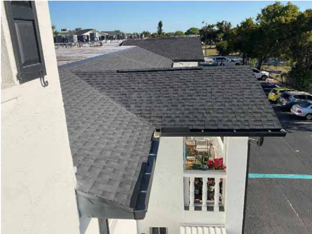
Bldg A Roof
