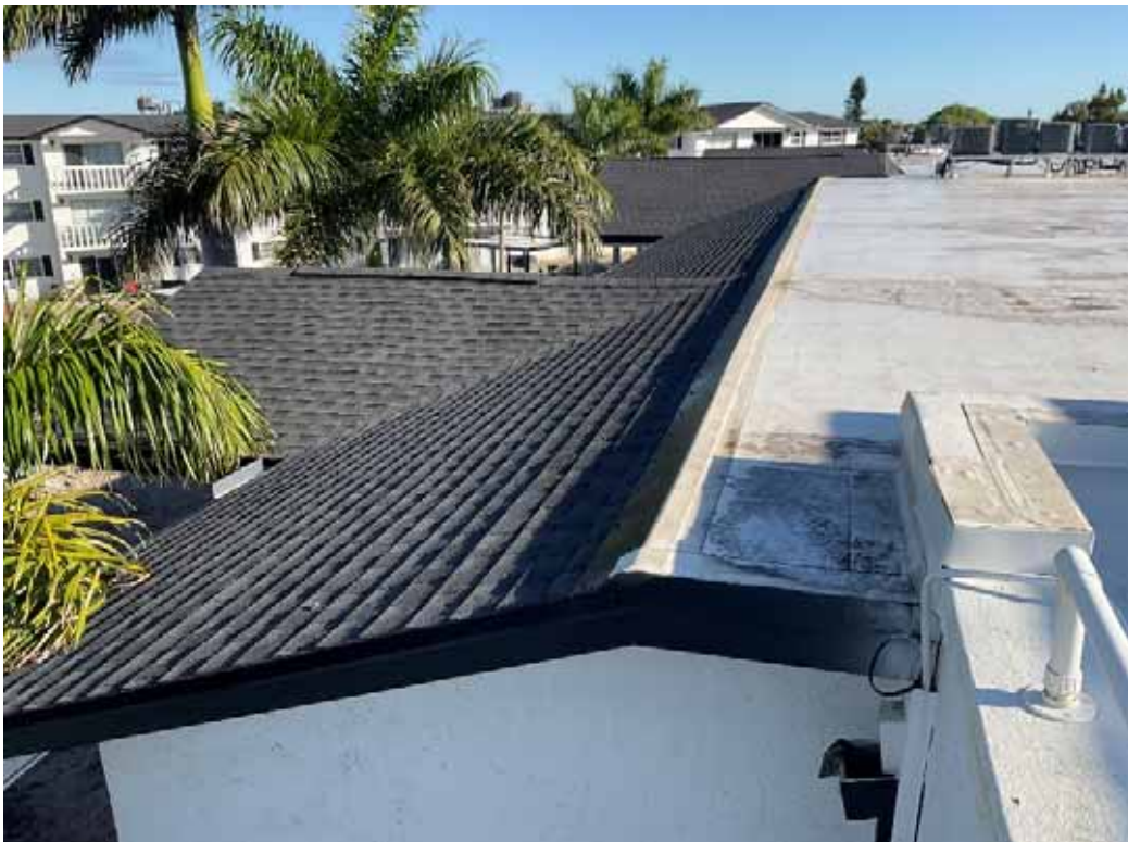
Bldg A Roof
