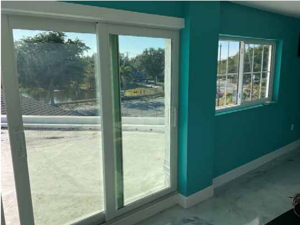
Bldg A Windows & Sliding Doors - Card Room
