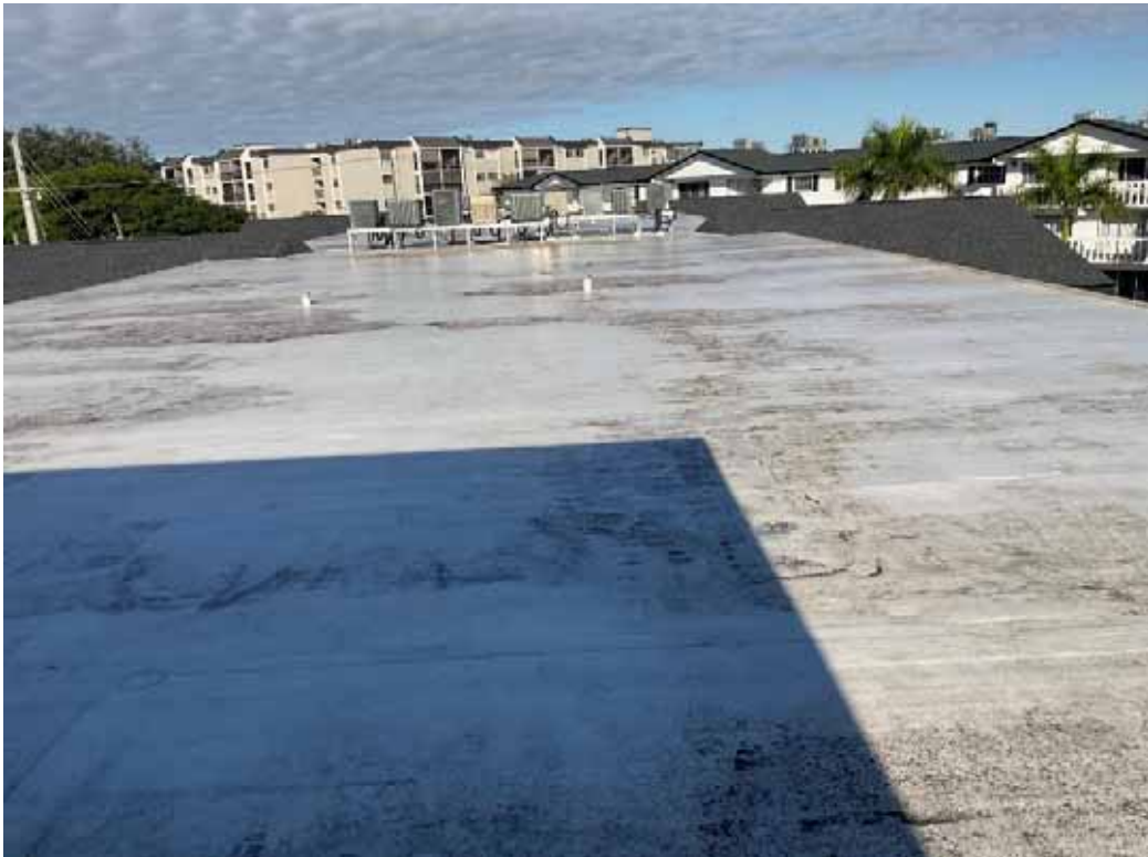
Bldg A Roof
