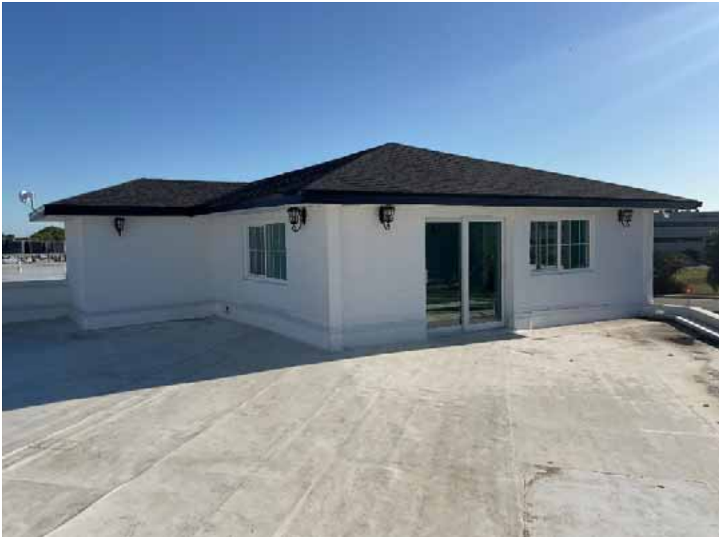
Bldg A Card Room Exterior (1 of 2)
