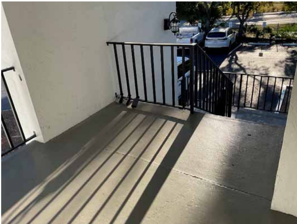
Bldg A Stairway
