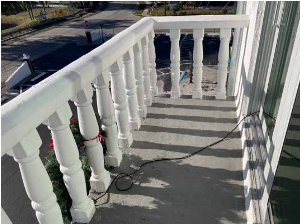
Bldg A Card Room Balcony (1 of 2)
