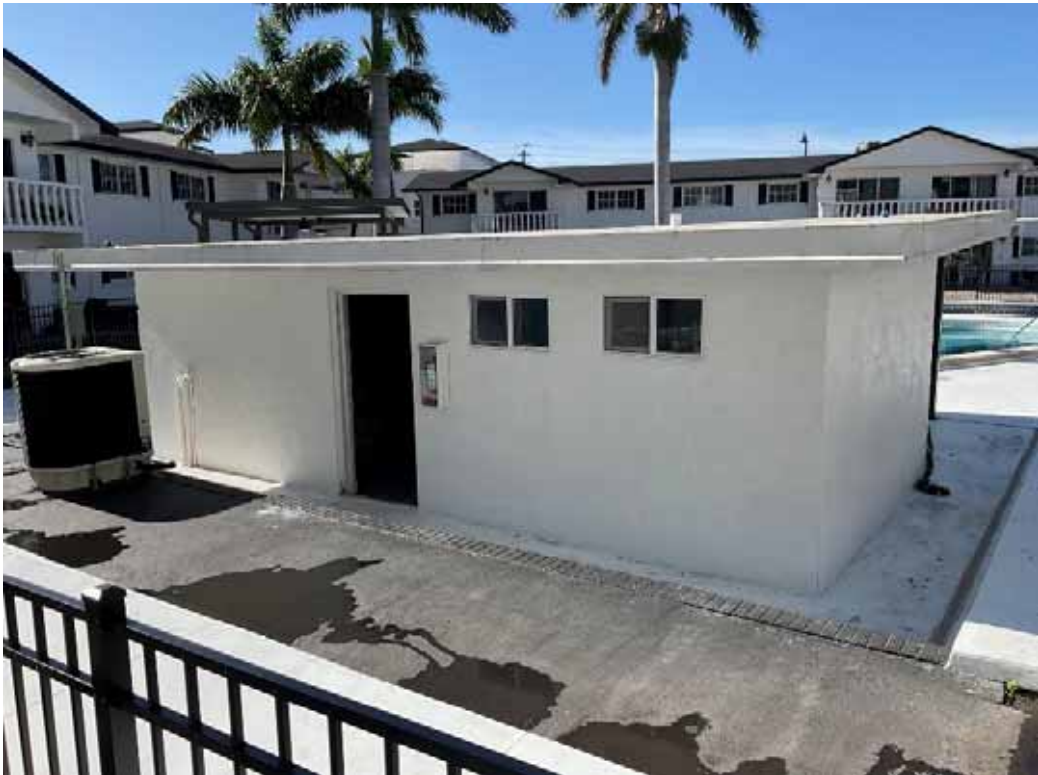
Pool Restroom Bldg
